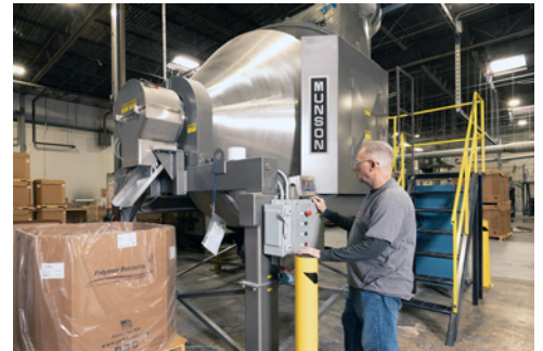
Operator programs mixing cycles at a frame-mounted control panel.
